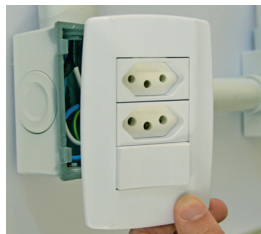
Figura 1 - Retire o interruptor
